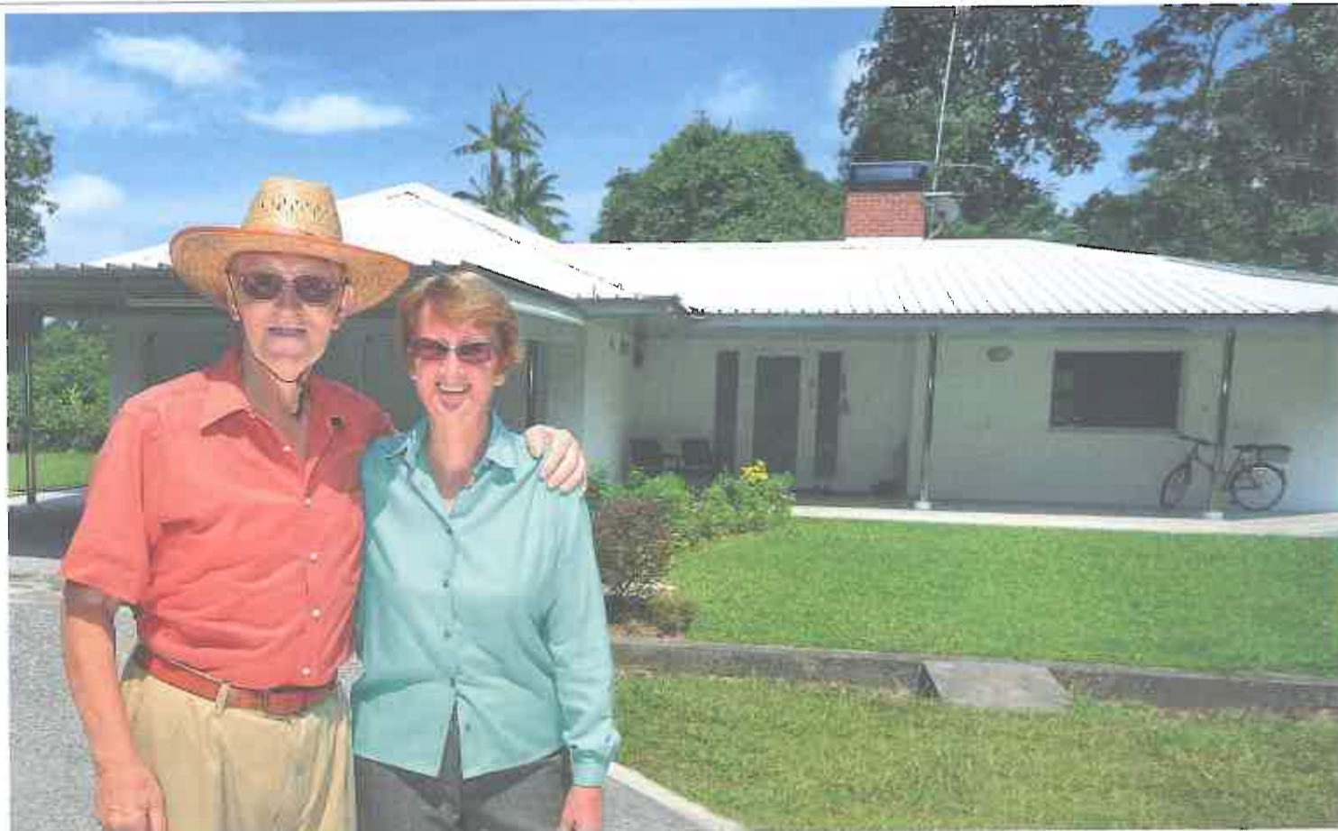
Harry Boswell and Stephanie Bacon in front of the Cooltek House in Melaka which they built in 2005. Air-conditioning the building 24 hours a day costs only RM2 a day
